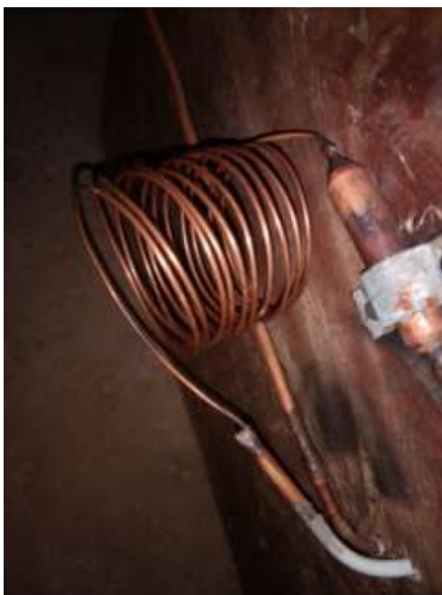
Fig. 4. capillary tube 2 Size: d= 0.04 -inch, L: 8 feet
